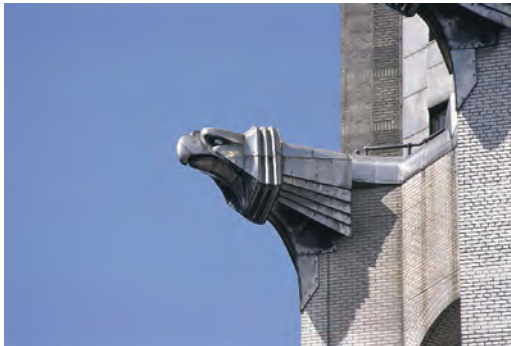
Chrysler Building , New York (1930), designed by William Van Alen Steel supported brick construction, stainless steel cladding on crown. Height: 318·9 metres, 77 floors.
